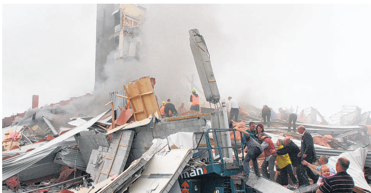
The Christchurch earthquake has forced many firms to reassess the seismic soundness of their buildings.
